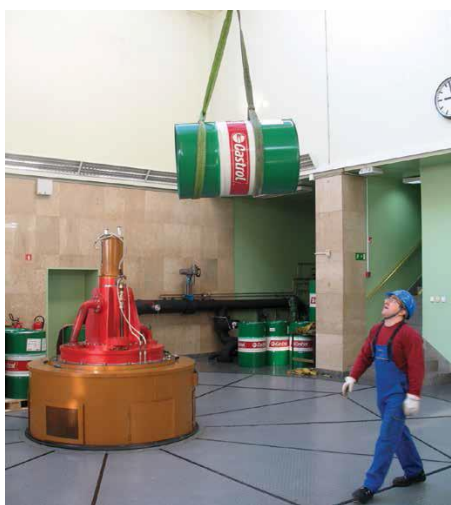
REPLACEMENT OF THE REGULATING OIL - GENERATOR 1 MARIBORSKI OTOK HPP
