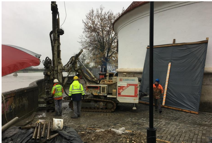
DRILLING FOR THE DRIVING OF AB PILOTS TO STABILIZE THE FLOOD PROTECTION WALL AT MIHELİČEVA GALERIJA IN PTUJ
