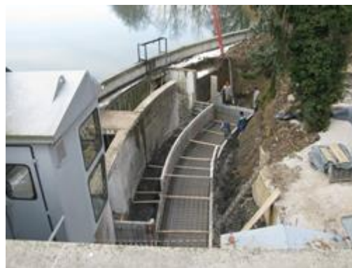
COMPLETION OF THE DISCHARGE SECTION AND CONSTRUCTION OF THE ADDITIONAL INLET CHANNEL THAT WILL PROVIDE CONTINUOUS WATER FLOW
