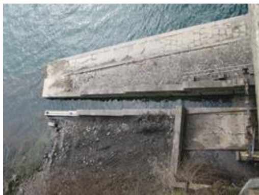
COMPLETION OF THE DISCHARGE SECTION AND CONSTRUCTION OF THE ADDITIONAL INLET CHANNEL THAT WILL PROVIDE CONTINUOUS WATER FLOW
